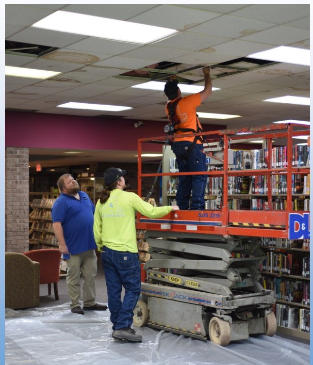
Workers Replace 1 of 5 HVAC Units
