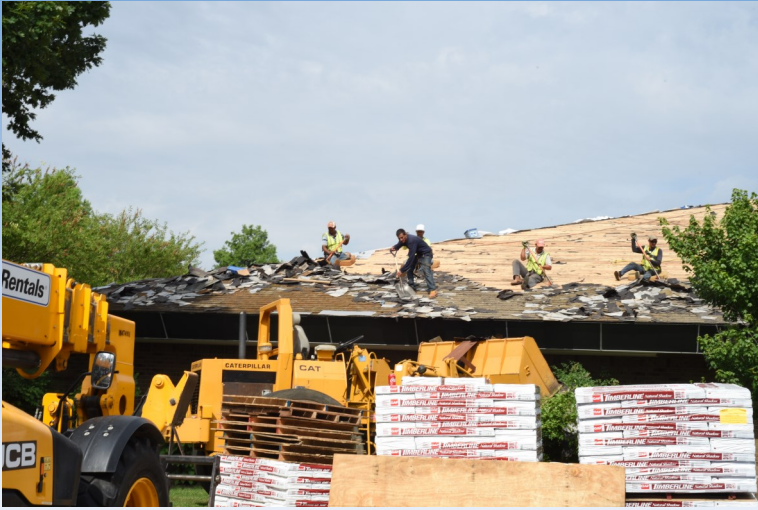
Replacing Shingles & Reinforcing Structure
